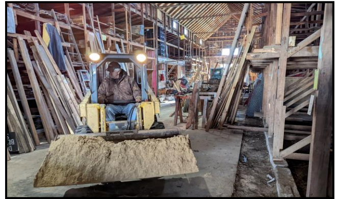
Jim Hunter operating the skid steer and bringing in the sand
